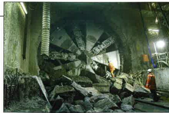
Londres, Crossrail : premier percement / London, Crossrail : first breakthrough.
